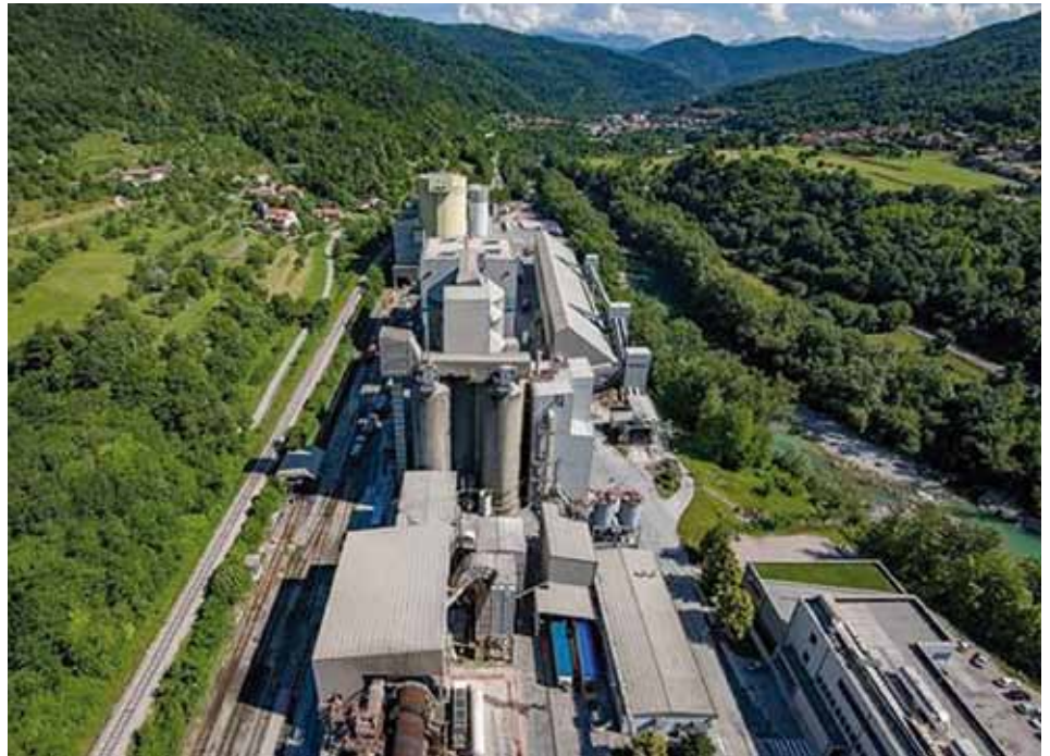
Cement factory Salanit, Anhovo (Slovenia)
